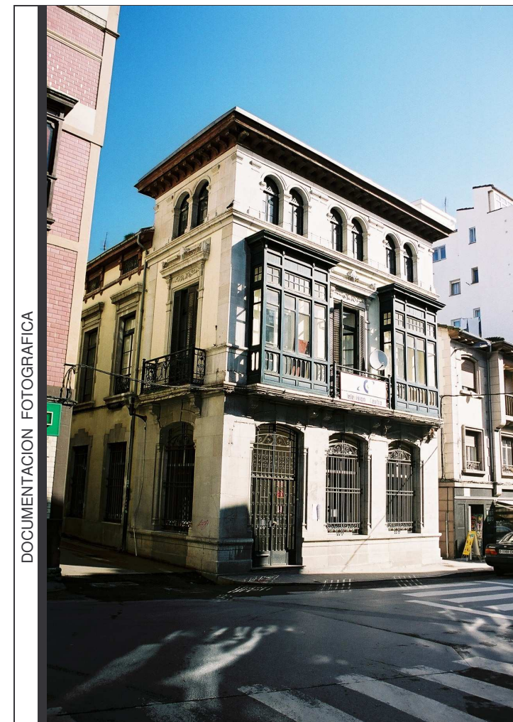
Fachada principal, a C/ Celleruelo
